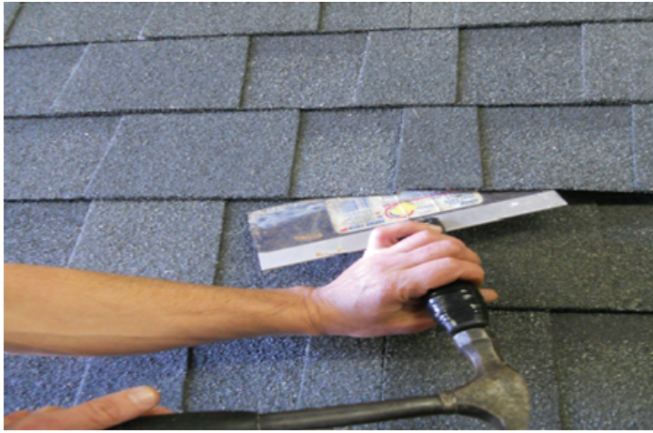
Figure 13. Lifting Shingles for Installation of Heating Panels
