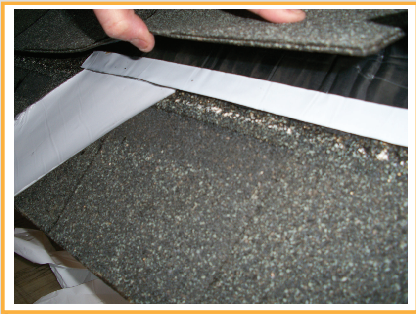
Figure 11. Removing Release Liner
